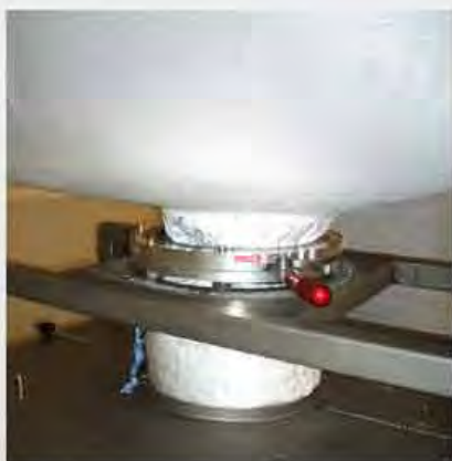
12" (305mm) Iris Valve on bulk bag discharge
