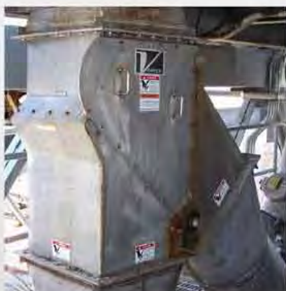
24" (610mm) straight line Seal Tite Diverter handling DDG
