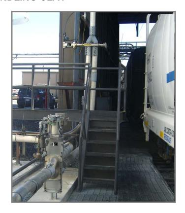
In addition to increasing efficiency of operation, the customer also desired flexibility in the routing of material to alternate locations within the facility. Specifically, the ability to convey to either the storage silos or directly into day bins located inside the plant from the railcar unloading system.
